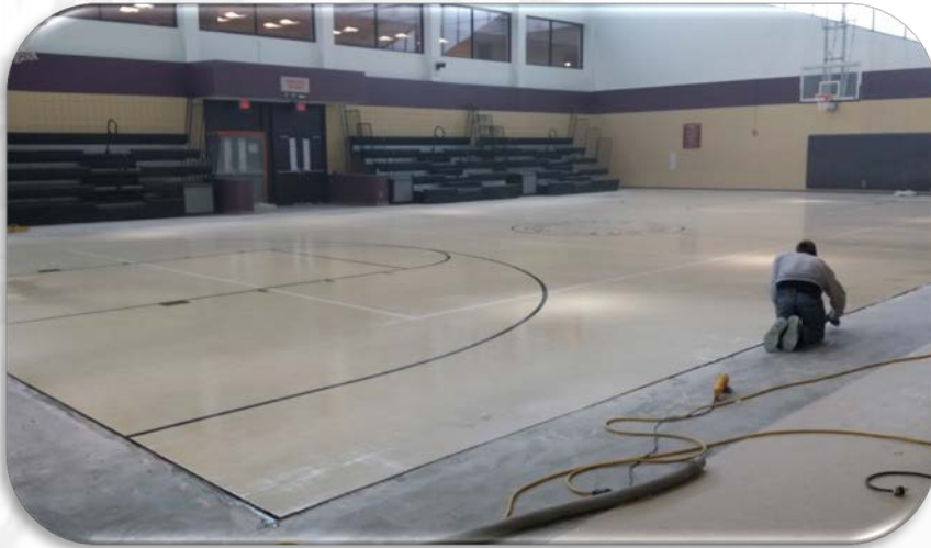
Treme Center Gym/Pool Repairs
