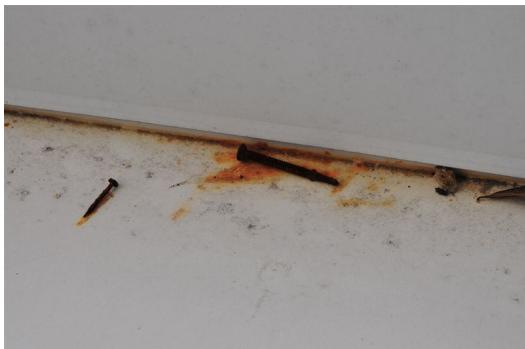
Figure 31. Rust spots on the roof panels caused by rusting screws left there by careless contractor workers.
