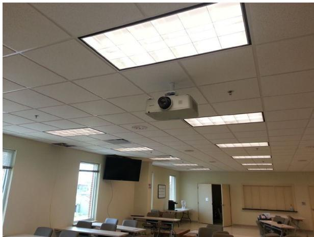
Figure 33. Ceiling mounted projector and 50 in. monitor in the background.
