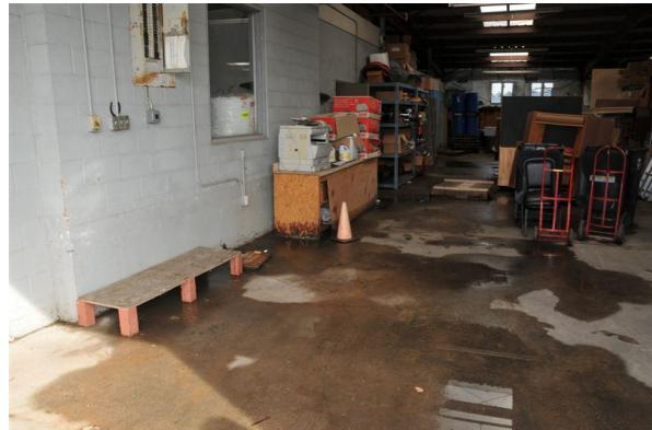
Figure 8. The waterline showed that approximately six to eight inches of water entered the middleshop.
