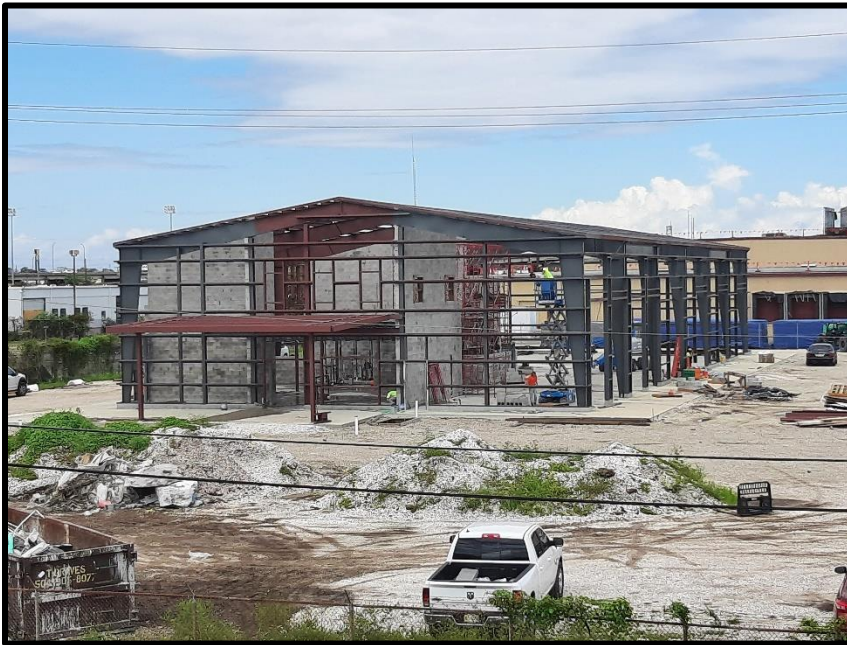
Figure 1: Ongoing Construction of the new EMD Building
