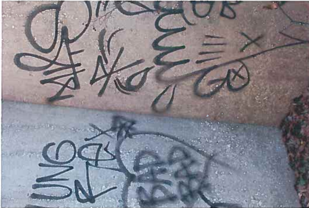
Condition Photo 6: Sidewalk and parapet/railing with graffiti sprayed with paint (northeast corner of Bridge Recall No. 102114 shown).
