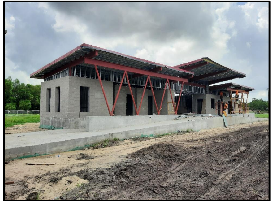
Figure 9: Current Construction of Village de L'est Multi-purpose building
