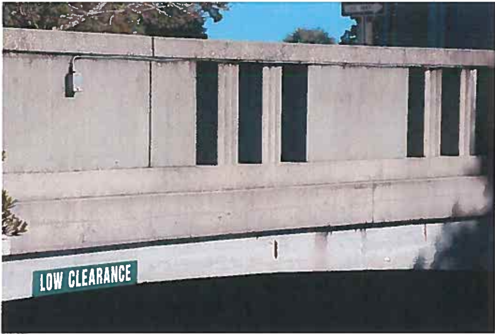
Condition Photo 16: Spalled and delaminated concrete on underside of Recall No. 102234 and sides of rigid frame.
