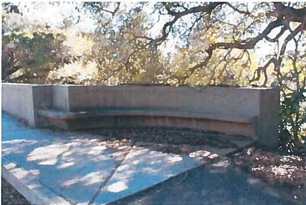
Character-defining Feature Photo 4: Aesthetic treatment seen in integrated benches walls (Recall No. 102113 shown).
