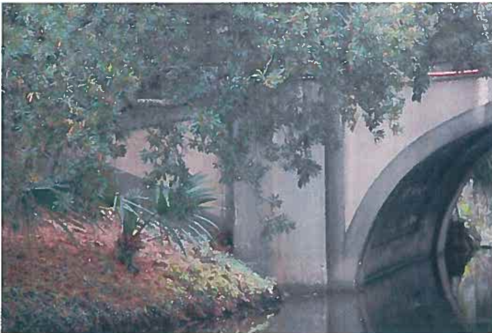
Character-defining Feature Photo 8: Aesthetic treatment seen in recessed panels in spandrel walls. (Recall No. 102227 shown).
