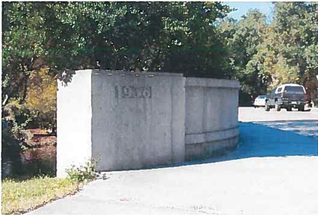
Character-defining Feature Photo 3: Design of reinforced-concrete superstructure with integrated curved wing walls and aesthetic treatment seen in bold font in Art Deco style letters in the concrete endposts and crowned parapets/railings (Recall No. 102234 shown).
