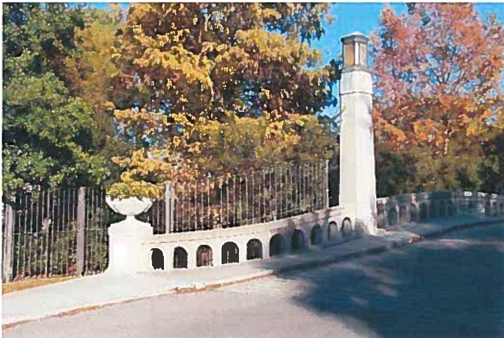
Character-defining Feature Photo 6: Aesthetic treatment seen in curved railing with arched posts, integrated lamp posts with decorative Classical Revival style lantern, and decorative endposts with integrated concrete urns (Recall No. 102227 shown).
