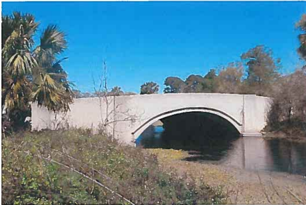
Character-defining Feature Photo 1: Design and construction of a closed-spandrel, reinforced-concrete arch with integrated curved wing walls and recessed arch ring (Recall No. 102237 shown).
