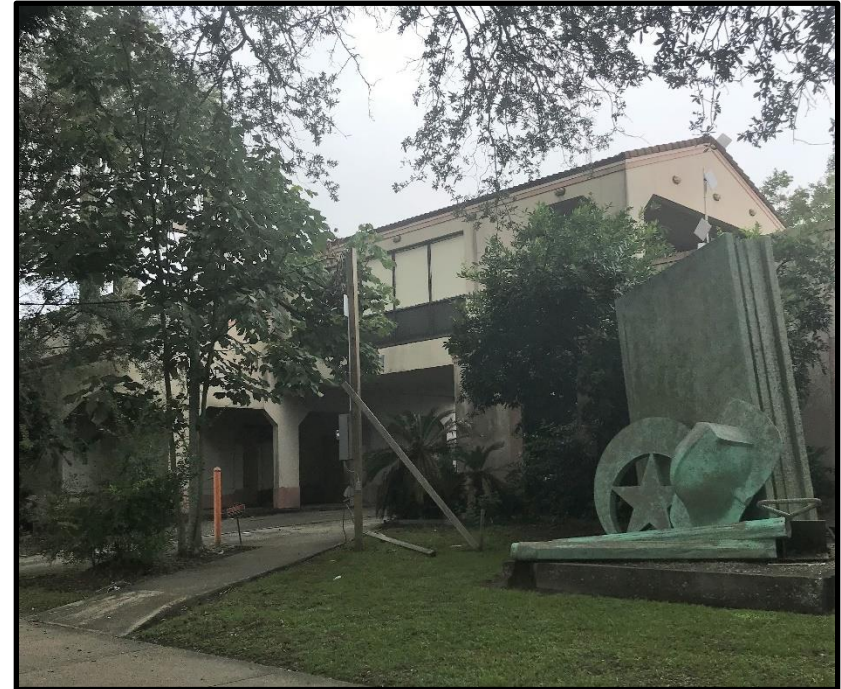
Figure 6: Front Façade of the existing NOFD Headquarters
