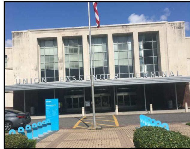
Figure 2: Front Façade of UPT Building
