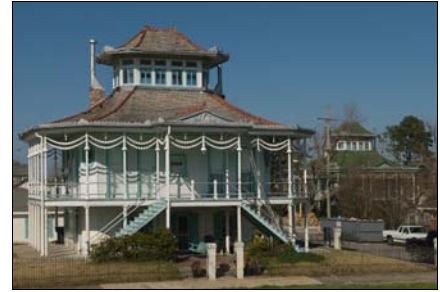
The Doullut houses were constructed to resemble steamships
