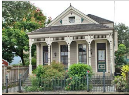
Shotgun houses show various stylistic details, featuring stock millwork of the time
