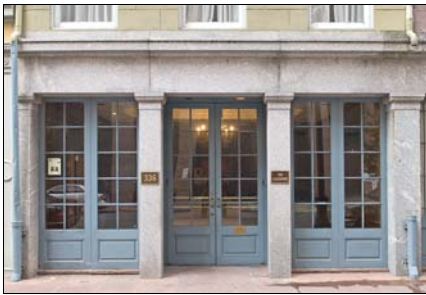
Storefronts with granite posts and lintels are common in the District
