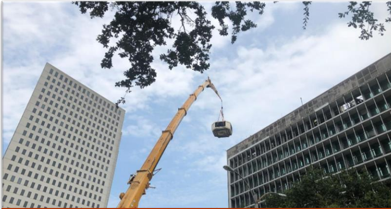
City Hall MEP (Supply Side) Upgrades
