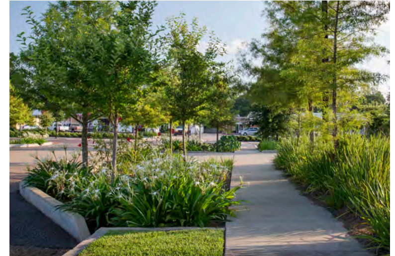
Urban bioretention cell, Alexandria, LA
