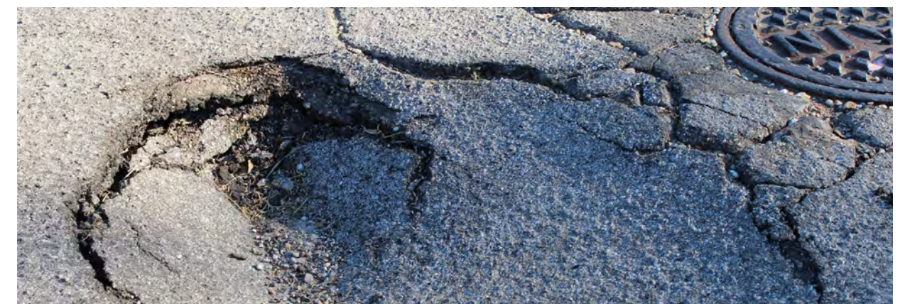
Subsidence-caused Street Damage on Owens Boulevard
