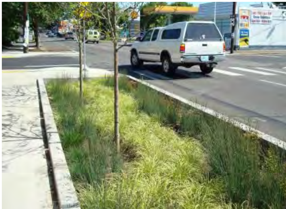
Urban bioretention cell
