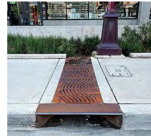
Grate connecting to street bioretention cells
