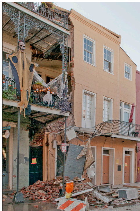
Although the façade of this c. 1800 building was recently repaired, the building's structure did not receive required maintenance. This resulted in a collapse, pedestrian hazard and the ultimate loss of the entire building.
