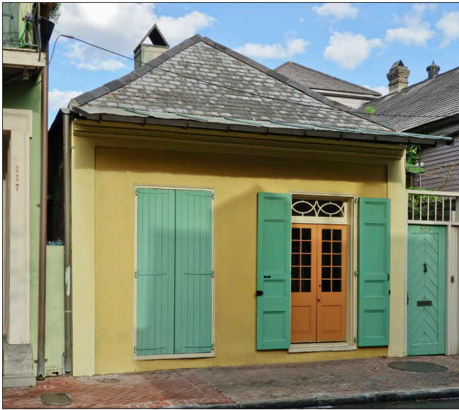
This 2-bay, Creole cottage has a hipped slate roof with a projecting abat-vent. The French door is topped by a transom, and the solid shutters with strap hinges are typical of the Creole style.
