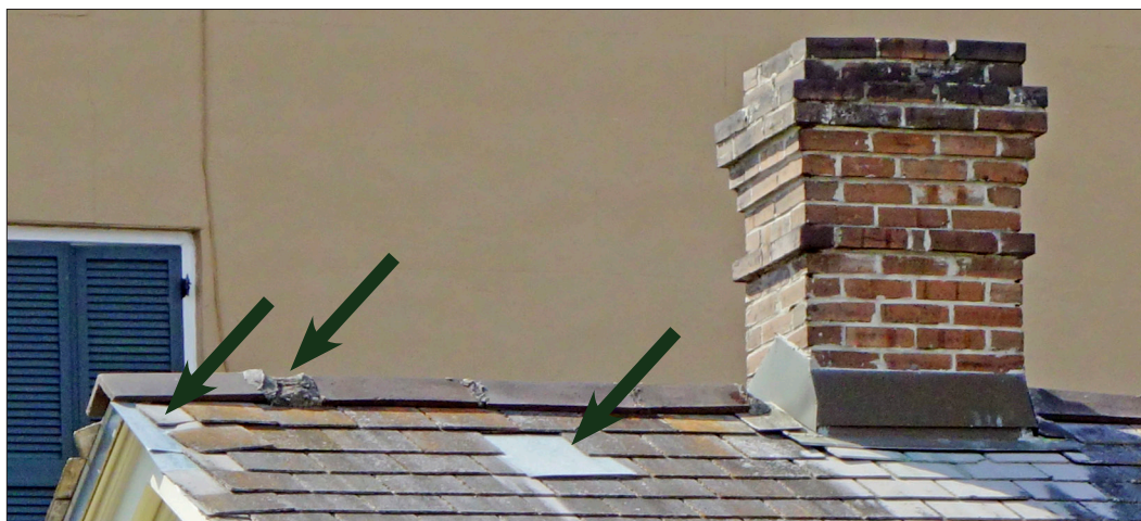
Prior patching is evident in multiple roof locations. Note the poorly executed expanded ridge joint repair of the ridge tile.
