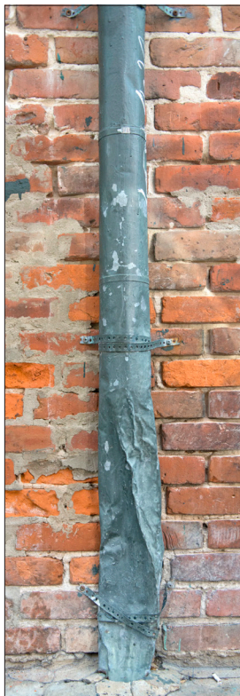
The crushed downspout is impeding water flow.
