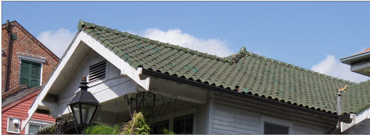
The terra cotta at this roof includes a green glaze. Also note that specialty shapes are used along the ridge cap and hips, and exposed metal flashing is located in the valley.
