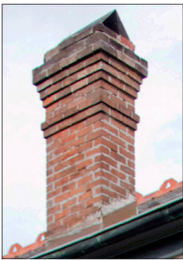
Chimney with "V" cap (left), and terra cotta chimney pots (right).
