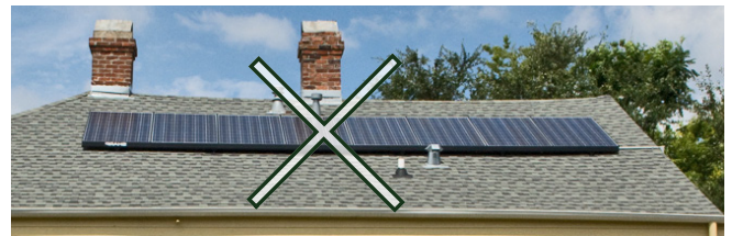
This solar collector is highly reflective making it more noticeable and visually dominant on the roof surface.
