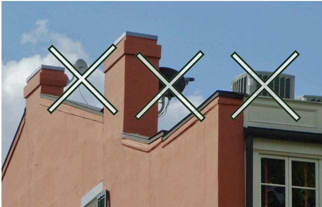
This roof includes a visible air compressor unit and two television dishes. Roof mounted equipment should be located to minimize visibility from all locations.
