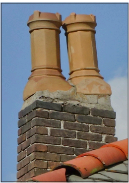
Chimney with "V" cap (left), and terra cotta chimney pots (right).
