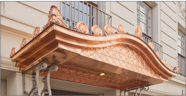
Sheet metal such as copper may be formed in a variety of shapes with different patterns. This entrance hood will naturally acquire a patina, turning green over time.
