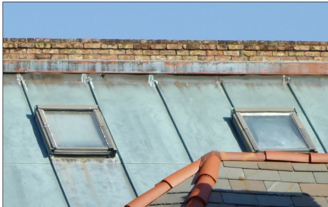
These skylights have a low profile and are located at least 12-inches below the top of this standing seam copper roof.
