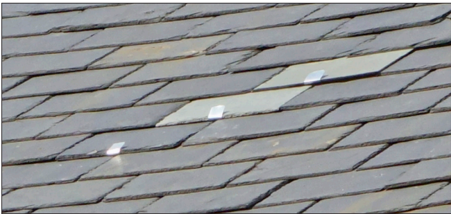
Metal hangers often are used to secure dislodged slates or replace individual slates.
