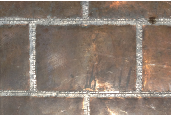
For a low-sloped or flat roof, copper sheets can be soldered together for a weather-tight surface.
