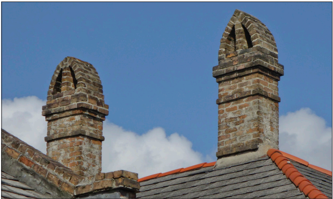
These chimneys have "Bishop Cap" tops formed with bricks.
