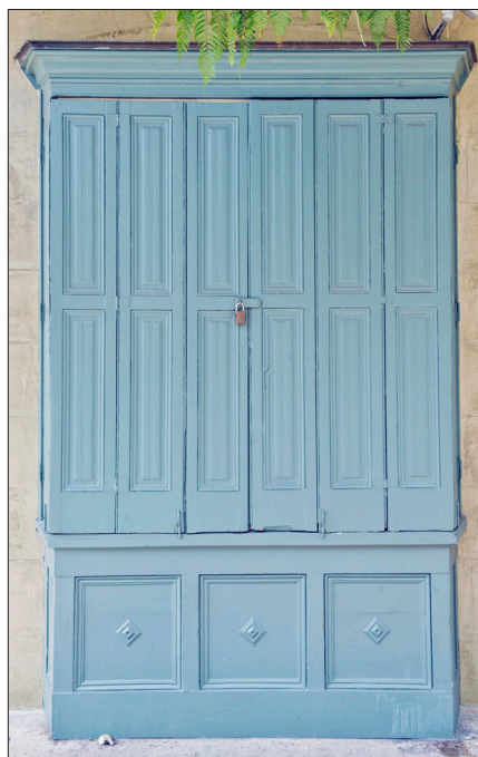
The wood-paneled blinds covering the vitrine in the left photograph can be unlocked and folded back to allow visibility of merchandise during store hours. The right photograph shows the paneled blinds folded open at a similar window.
