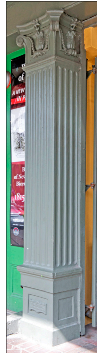
Fluted Cast Iron Pilaster With Paneled Plinth
