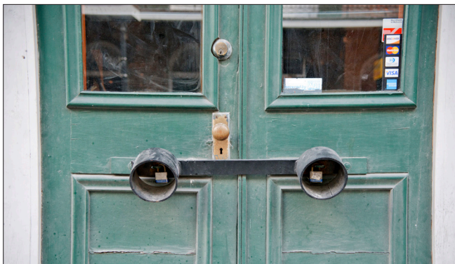
The padlocked bar extending across the doors is removed when the store is open. The bar provides added security from a potential intruder who might consider pushing the paired doors open.
