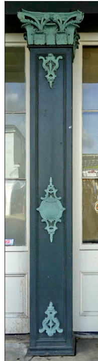
Cast Iron Pilaster With Applied Ornament
