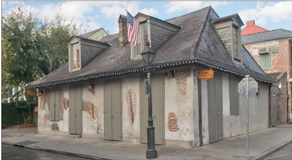
Lafitte's Blacksmith Shop, a National Historic Landmark, was built in the Spanish Colonial period with the dormers added later. Originally a shop was located in the right half and a residence in the left half. The interior spaces have been combined, and the building is now used as a bar.
