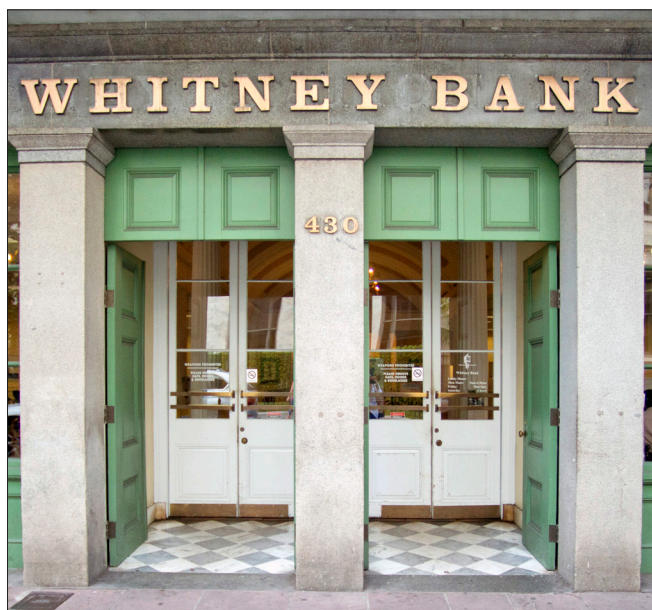
The interior pair of doors creates a vestibule. When the wood paneled shutters are closed, the shutters provide enhanced security from intruders. When the shutters are open during operating hours, the interior doors allow natural light to enter the business.
