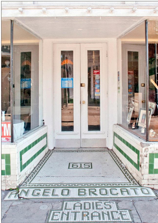
The alcove ceiling is beadboard and the ceramic tile flooring includes the street number and former business name.
