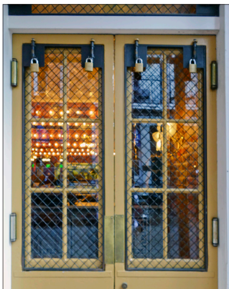
The padlocked bar extending across the doors is removed when the store is open. The bar provides added security from a potential intruder who might consider pushing the paired doors open.
