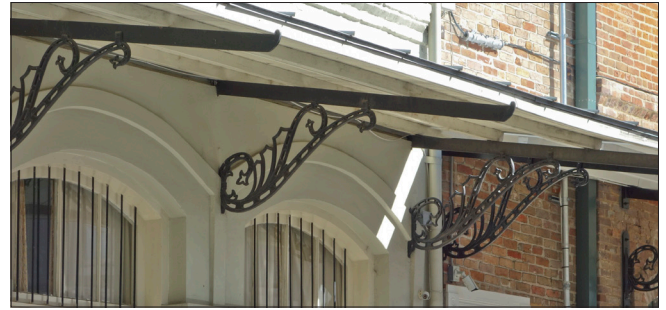
This canopy provides protection for pedestrians along the sidewalk. It has a standing seam metal roof and is supported by decorative metal brackets.
