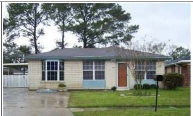
This home in Jefferson Parish has permanent shields sealing the space under the windows.
