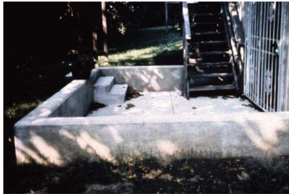
This low floodwall does not have any openings, so it provides protection even if no one is home.
