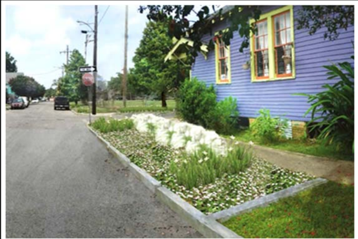
Rendering of how street corners would be altered to convert impervious surfaces to rain gardens
