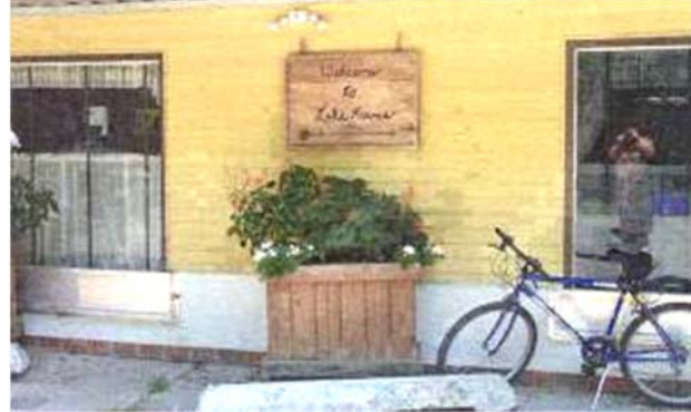
This dry floodproofed building in Mandeville had the walls waterproofed and removable shields placed in the windows.
