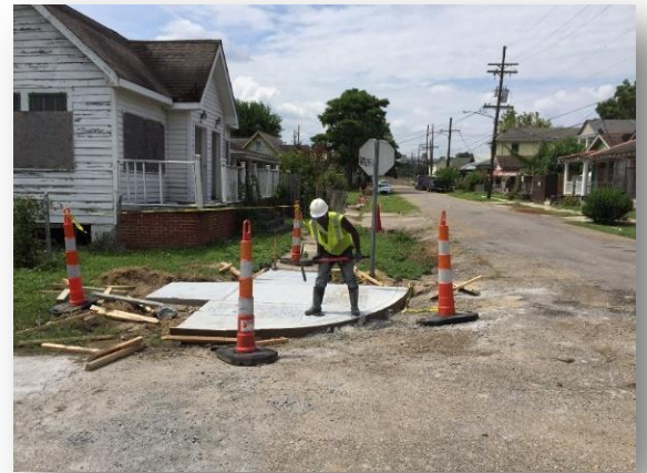
Non-Paving Incidental work includes installing American with Disabilities Act-compliant curb ramps at intersections.
