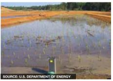
Constructed wetlands are artificial ponds planted with aquatic plants that are used to treat waste water, and have been successfully utilized in several municipalities throughout the U.S. The New Orleans Sewerage and Water Board is developing a project to restore degraded wetlands as a way of treating effluent from the East Bank wastewater treatment plant. If successful, this project could obviate the need for expensive infrastructure investments.
