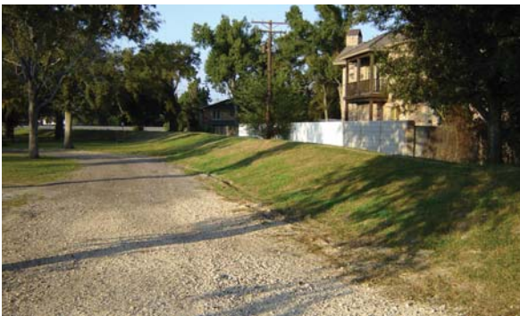
Berm surrounding a neighborhood park in suburban Jefferson Parish which has been re-designed to store stormwater in the event of a heavy rainfall.
