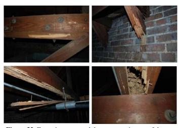
**Figure 32.** Extensive structural damage to attic area of the Cita Dennis Hubbel Branch of the New Orleans Public Library remaining from a termite infestation remediated in 2005.
