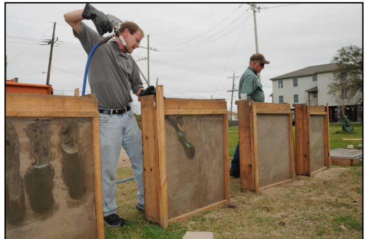
Figure 47. Timmy Madere demonstrates best practices for a liquid perimeter termite treatment when rodding.
