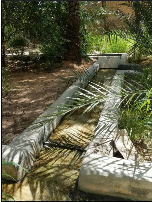
Figure 9. A water canal made of concrete within the oasis.
