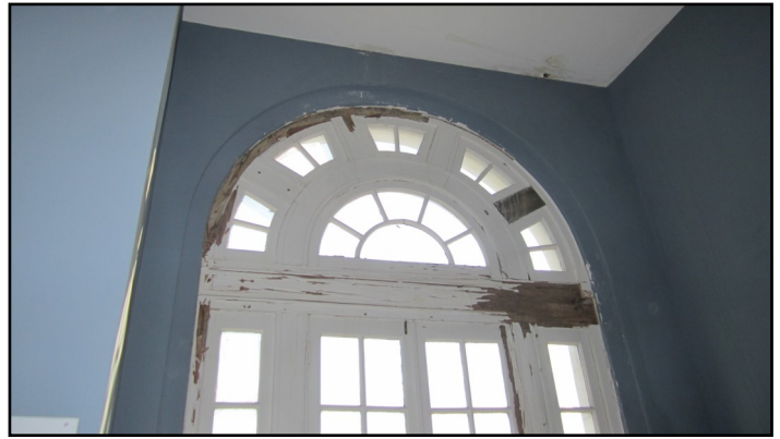
Figure 49 . Termite damage around a window frame in a museum in Mobile, AL.
