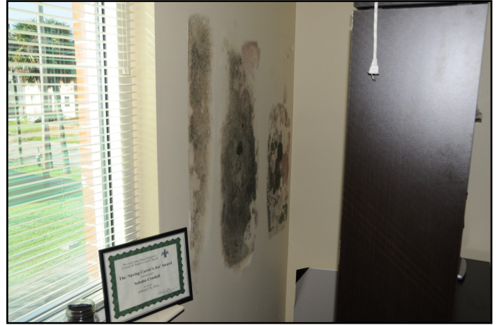
Figure 40. Mold growth behind a book shelf in an office of the new administration building.
