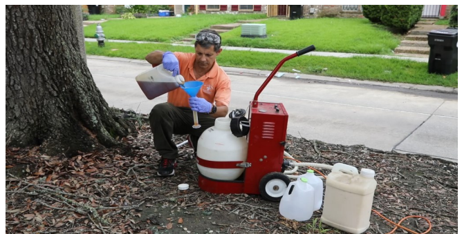
Figure 57. Measuring foaming agent to calibrate unit to produce 15 gallons of foam per gallon of solution.
