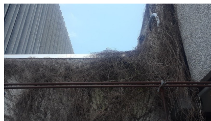
Figure 31. A rodent entry point at the Police Headquarters. Vines were killed and removed and the building fascia replaced.
