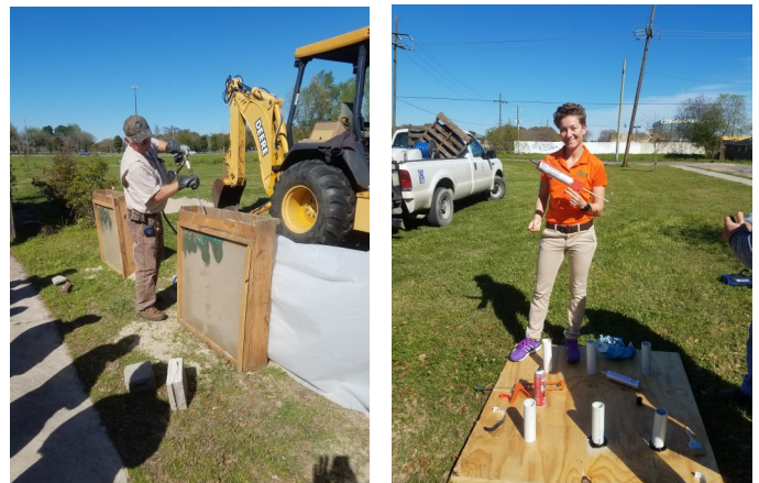
Fig. 61. Milton Schleismann (left) demonstrates best practices for rodding techniques with a liquid termiticide. Holly Beard (right) demonstrates the use of Polyguard sealant around plumbing penetrations to help prevent termites from entering a home.
