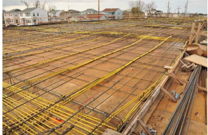
Figure 46. The cables were visible for pre-tensioning the slab for the second floor on 12/9/2010
