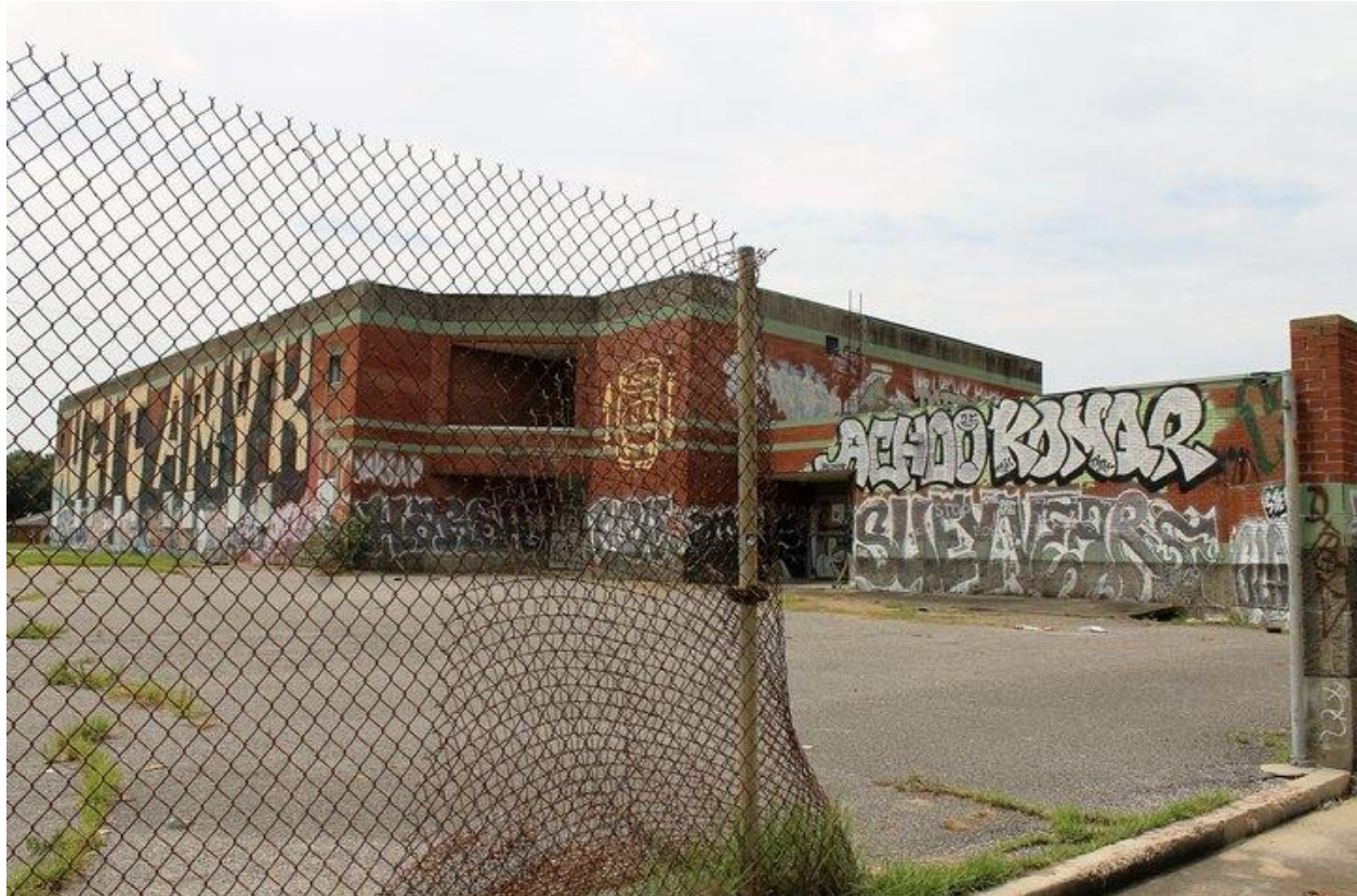
Figure 2. Moton Elementary School now vacant. Source: Huffington Post
