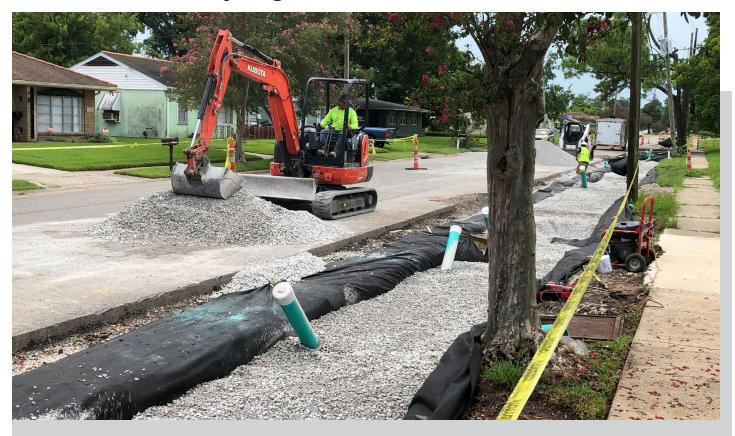
**Description:** A critical "gray-green" infrastructure feature of the Pontilly Neighborhood Stormwater Network is the addition of bioswales. The construction (above) shows the excavation of the street and connection of pipes that will collect and drain water during a rain event. Complete construction (below) will feature native vegetation that can thrive in Louisiana's subtropical climate.
