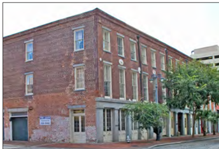
Buildings are typically set on the front lot line
