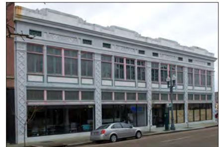
710 Baronne Street incorporates large storefront display windows
