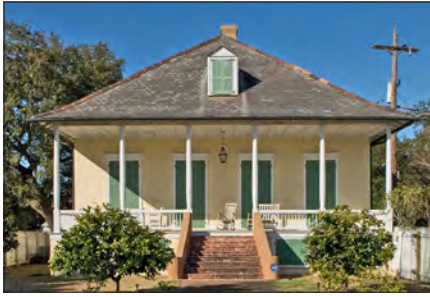
The Lombard Plantation House was built before Bywater was subdivided
