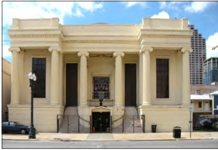
The Scottish Rite Temple is a distinctive building in the District.
