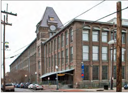
The Maginnis Cotton Mill, built 1882, was recently converted into residences
