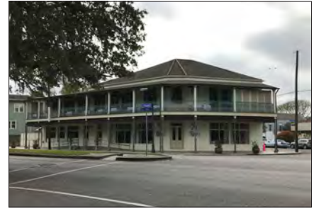
The Saux Building was constructed as a coffeehouse in 1859.
