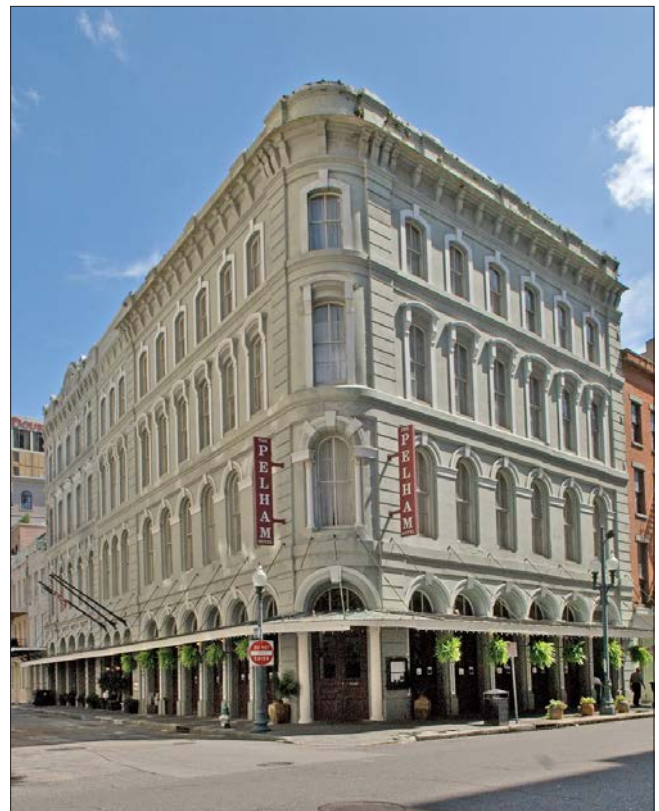
A flat or low-sloped roof is located behind the parapet and bracketed cornice.
