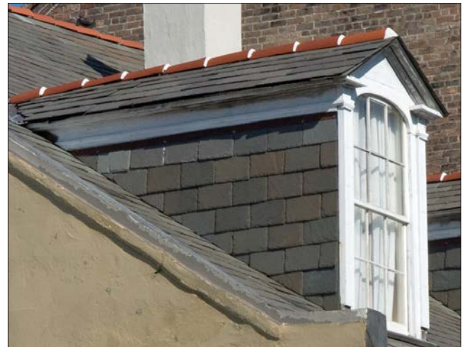
This gable roof dormer is appropriately located, proportioned and detailed for the building and include slate cheek walls. Spanish tile ridge caps should be retained.
