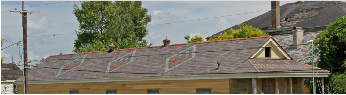
This distinctive slate roof with diamond patterns, terra cotta ridge caps, and Chinese caps are being retained as part of the rehabilitation project.
