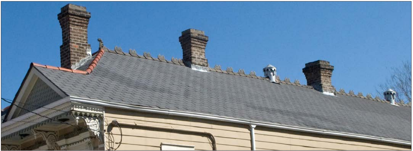
Ridge caps are located along the roof hips, cresting is along the top ridge and a finial is found at the end of the main roof gable. Chimney placement reflects the internal organization of the residence and Chinese caps provide roof ventilation.
