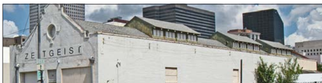
Roof monitors are more typically found on commercial buildings and often provide interior light and ventilation.
