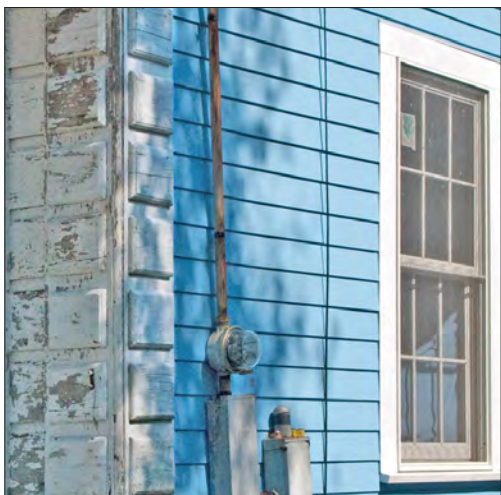
The side elevation has been covered with vinyl siding. The appearance is much flatter particularly at the windows.
