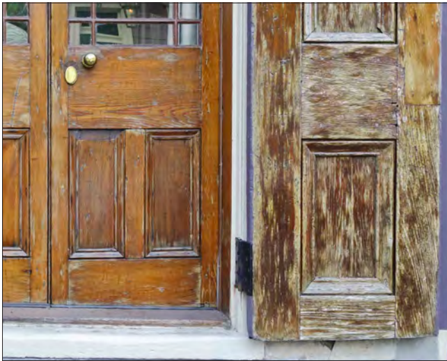
Semitransparent stains and varnishes are not recommended by the HDLC because they tend to deteriorate quickly in New Orleans' climate, leaving wood exposed and vulnerable to deterioration.
