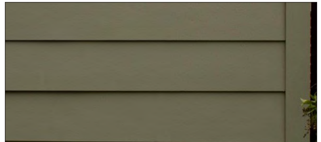
Fiber-cement siding material is a good economical alternative for new construction or an addition to a historic building. It can be painted to match the existing paint scheme.
