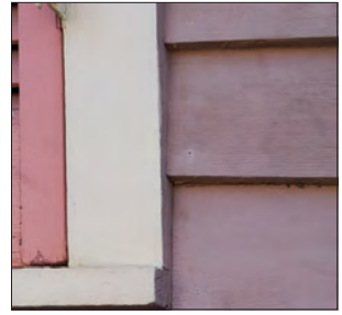
Siding should not extend past face of window trim. The window should also have a sill.
