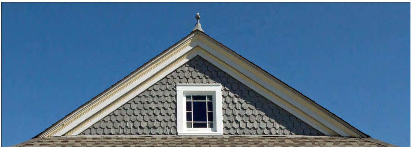
Decorative wood shingles are most often found in the front gables of residential buildings in New Orleans.
