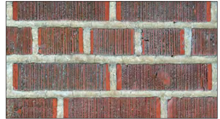
Wire Cut Brick – A dense, fired-clay, regularly shaped building component; with a ridged surface; used primarily in 20th century building walls.
