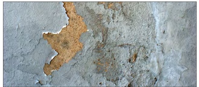
The peeling paint is likely incompatible with the stucco or caused by moisture. Loose and flaking paint should be removed and the cause for failure addressed before repainting.
