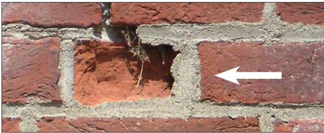
Spalling of the masonry surface – The center brick surface has spalled. The repointing mortar likely includes too much Portland cement and is harder than the bricks. The mortar should be removed and replaced with soft mortar.
