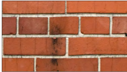
20th Century Brick – A hard, dense, fired-clay, regularly shaped building component; sometimes with a glazed surface; used primarily in walls, piers, foundations and exterior pavers.
