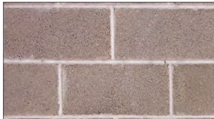
Concrete Block – A structural building material made by mixing water, cement, sand and aggregate, placing the mix in forms and hardening; commonly used for foundations, walls and piers.
