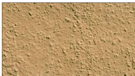
Dash Finish Stucco – Textured finish with pronounced aggregate at the surface.
