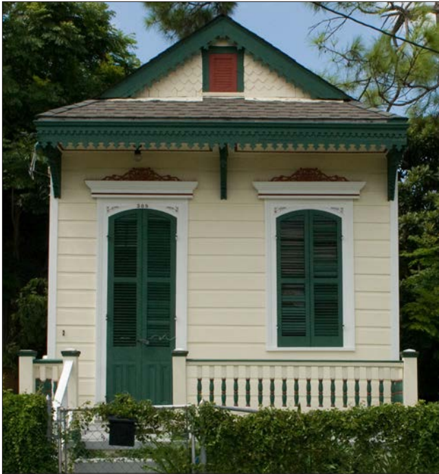
Fastening shutters and blinds provides protection from hurricanes and additional security.
