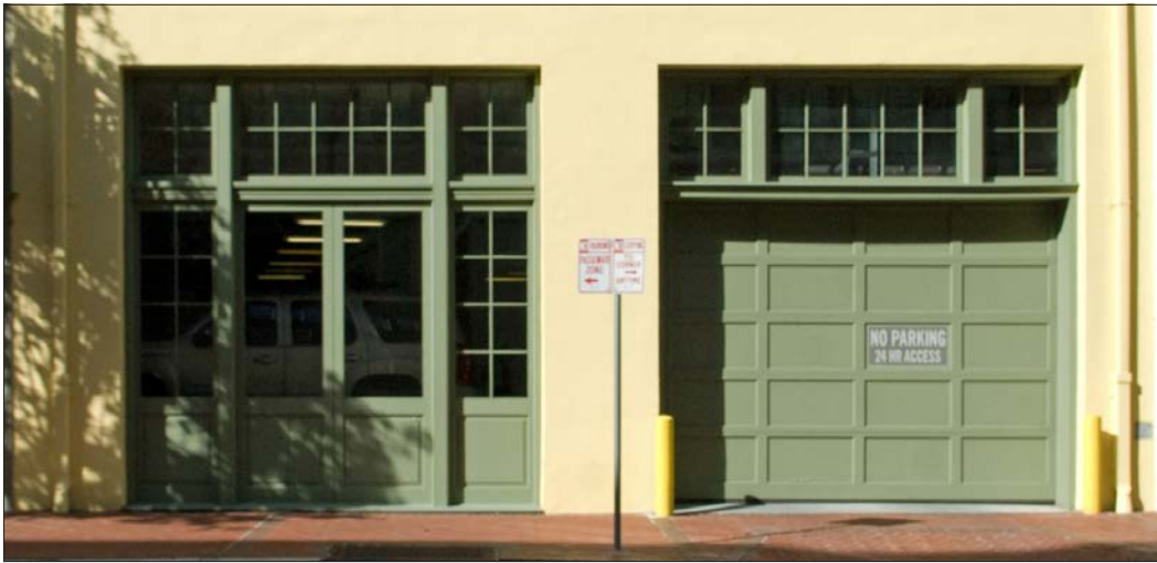
The former storefront opening to the right was modified for use as a garage. The historic transom window configuration matches the storefront to the left.
