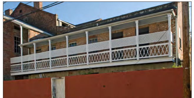
This service wing balcony includes a wood lattice privacy screen above the balustrade.
