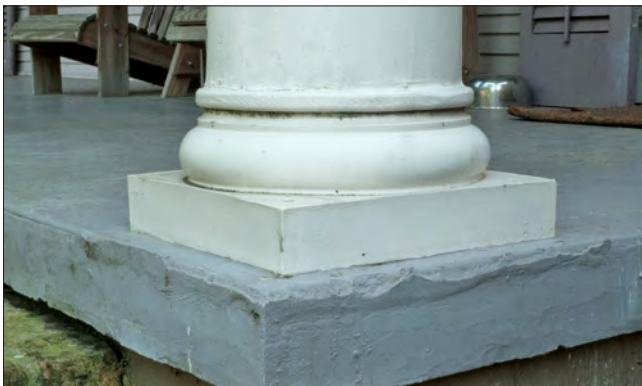
This porch column is wood, while the base is a composite.
