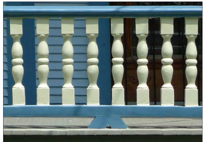
Turned wood balustrades are appropriate for most Italianate, Queen Anne and Eastlake homes. Historic balusters tend to be wider than many new, mass produced balusters.
