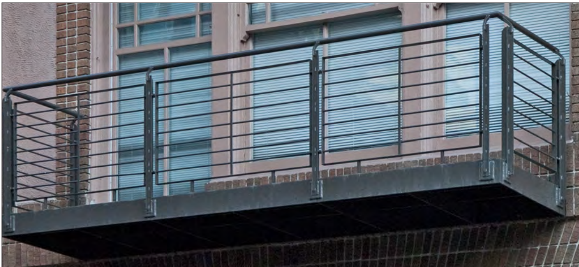
This balcony appears to “float” in front of the window and is fastened to the wall at the platform level.
