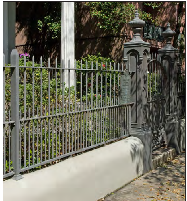
Wrought iron fences are often installed on low masonry chain walls less than 18” tall. Also note that the fence is relatively simple and made from narrow pickets, while the cast iron entrance gate posts are fairly ornate.
