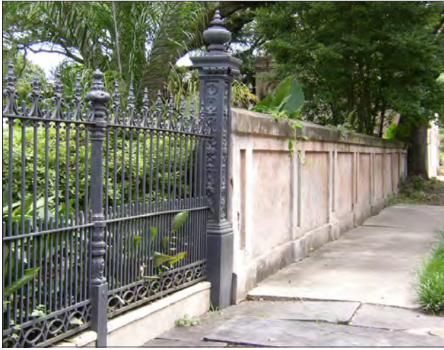
Cast iron fences often occur adjacent to masonry walls.
