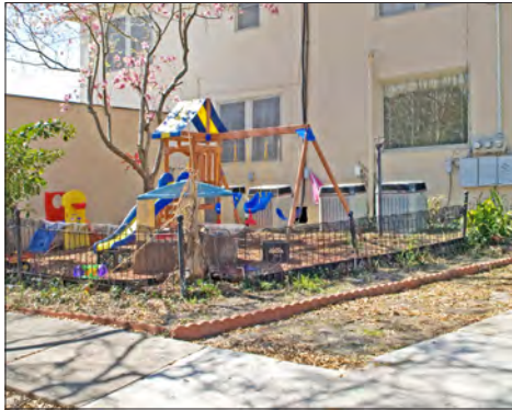
Shrubs and landscaping would provide screening of the play equipment and air conditioner units.
