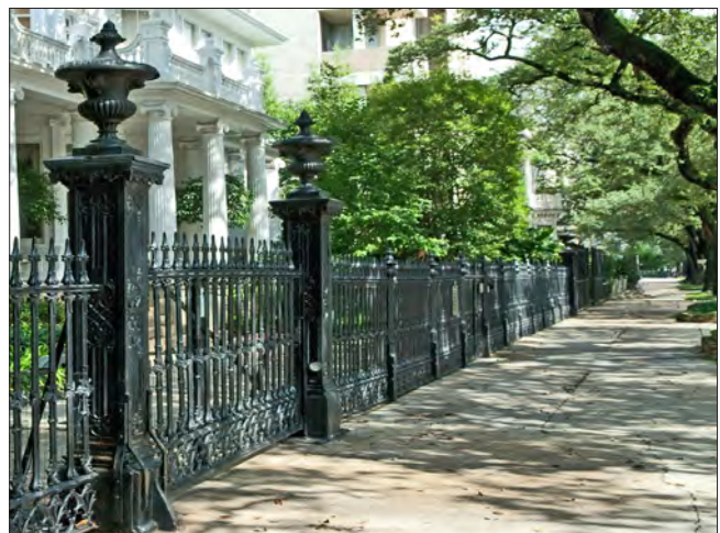
Most homes on St. Charles Avenue are set back from the street and include cast and wrought iron fences along the front property line.
