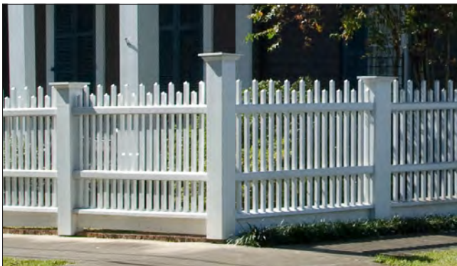
This fence includes 1” square wood pickets over a heavy bottom rail, supported by large wood posts – a style that was common in Greek revival homes.
