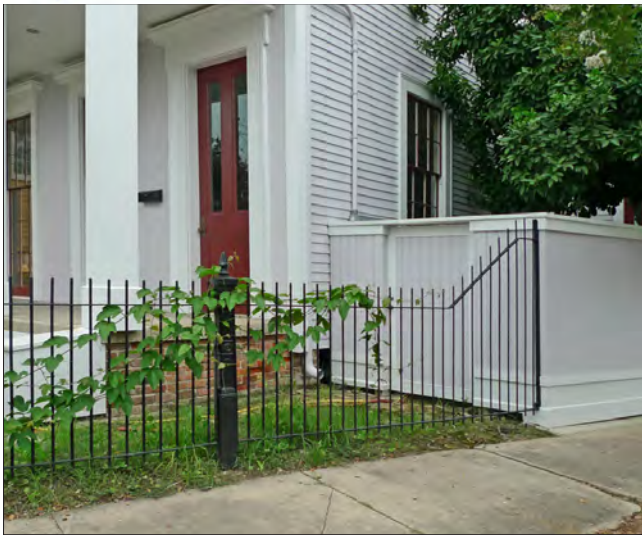
A smooth transition between a shorter front yard fence and a taller side yard fence may be installed with metal fencing as in the example above, but is typically unsuccessful in wood fencing.
