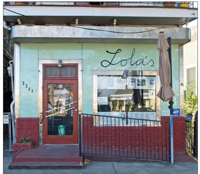
This building’s Vitrolite glass storefront is distinct from the residence above. It is historically significant and should be retained.
