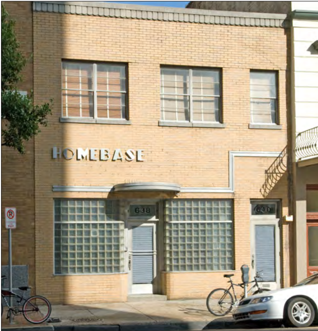
This Moderne building serves as professional offices. Similar to most commercial buildings, second floor windows appear “punched” through the masonry.
