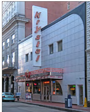
Neon has been used in the vertical blade sign as well as on the entrance marquee. At the blade sign, neon is used as an accent over individual channel letters. At the marquee, neon is used in the decorative stripes and central emblem.
