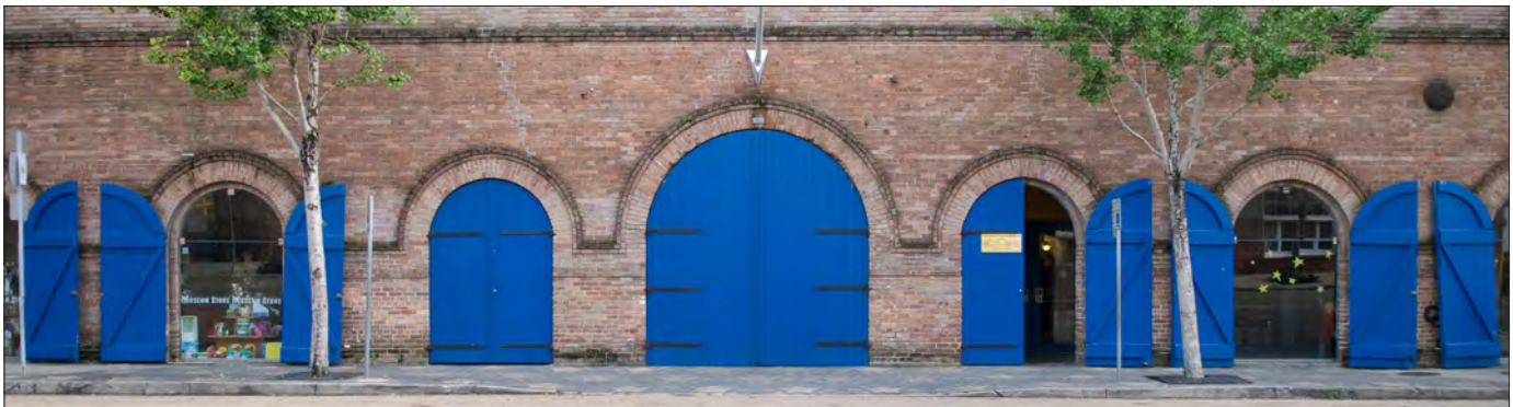
These historic solid shutters provide security for display windows and building entrances.
