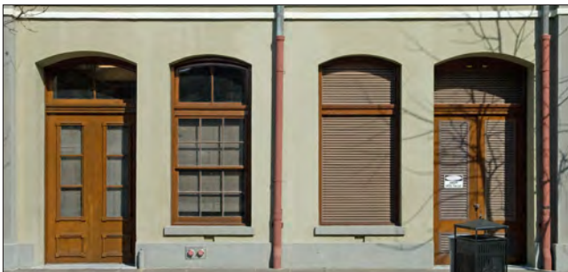
The rhythm of the storefront was maintained in the installation of the building equipment behind the louvered window and door.
