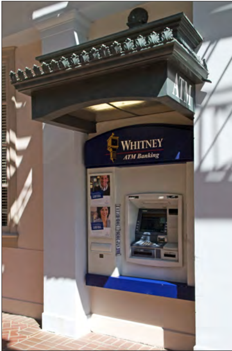
This ATM canopy was designed in a manner that complements the building's style and includes integrated down-lighting illuminating the immediate area.
