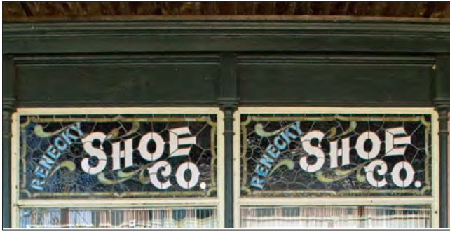
Stained and colored glass was sometimes used to create building signage. Historic signage should be retained if it reflects a historic building name, owner or early business.
