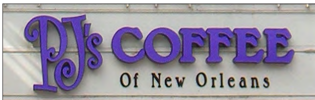
This internally individual illuminated channel letter sign is mounted flush to the wall and does not have an exterior raceway.
