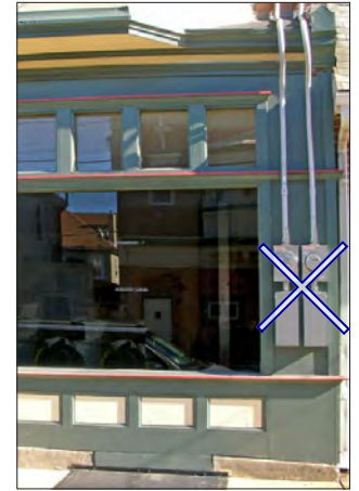
Restaurant ventilation equipment should not be mounted to the face of publicly visible elevations, nor should features like windows be removed for installation. Electric meters should not be located on the front elevation.
