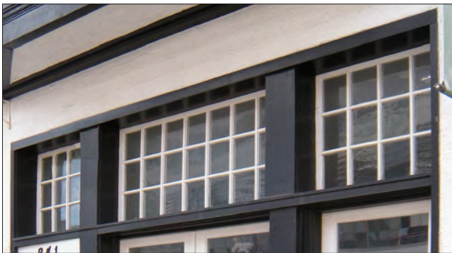
These multi-light transom windows provide additional light to the interior and add detail to the exterior storefront. Many transom windows were historically operable and allowed additional ventilation.
