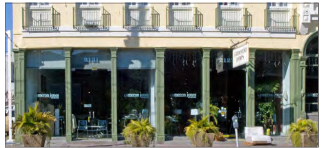
The large glass openings accentuate the cast iron columns.
