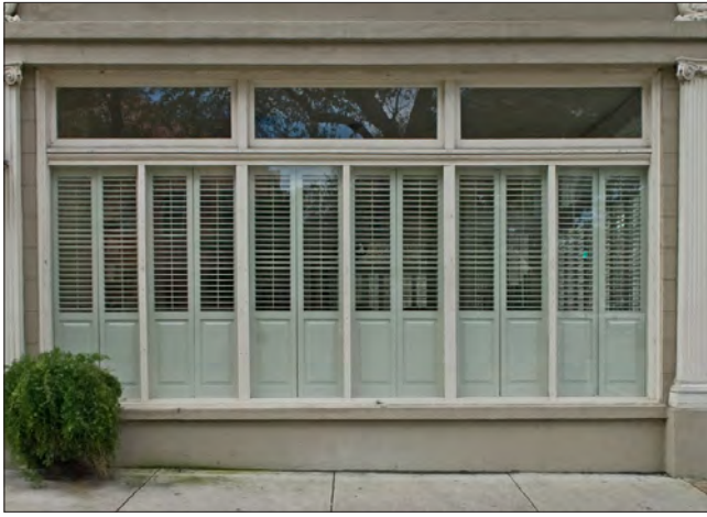
Blinds can be installed within storefronts or glazed openings to provide privacy while retaining historical integrity.
