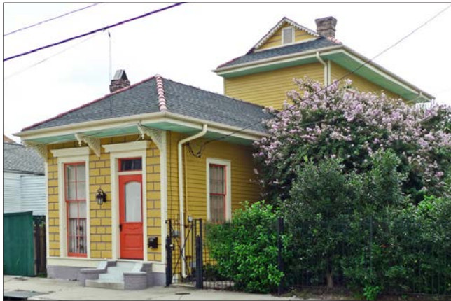
Camelback additions are typically found on wood-framed single and double shotguns.
