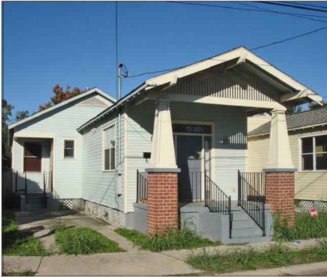
Trim and details at additions are often simpler than those at the main historic building. In this example, the rear addition has a simple rake board following the slope of the eave, but exposed rafter tails similar to the historic portion of the house.
