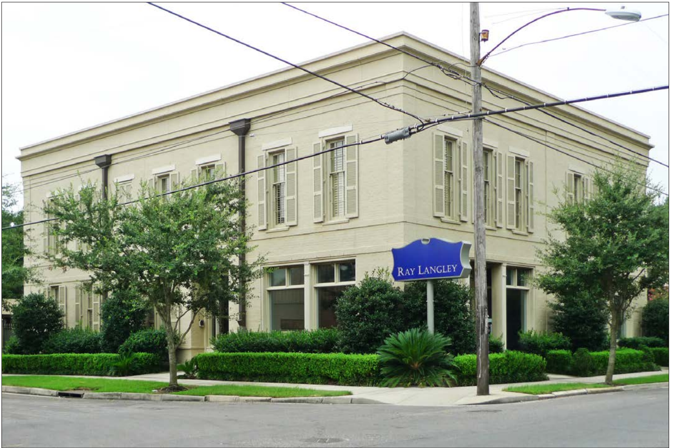
This is an example of a new building in a commercial corridor that utilizes traditional siting, proportion, scale, form, materials, fenestration, roof configuration, details, finishes and landscaping.
