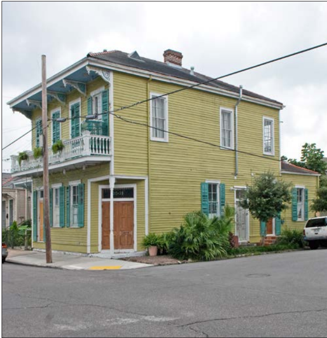
A 1-story addition has been added to the rear of this 2-story building. The scale, proportions, roof form, materials, window and shutter details are compatible to the historic building.
