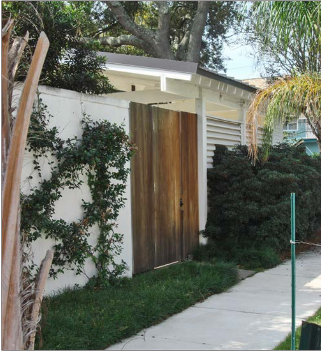
New secondary buildings should be complementary to existing historic buildings and the streetscape. This carport has a louvered side wall and roof structure with exposed rafter tails that resemble a neighborhood building.
