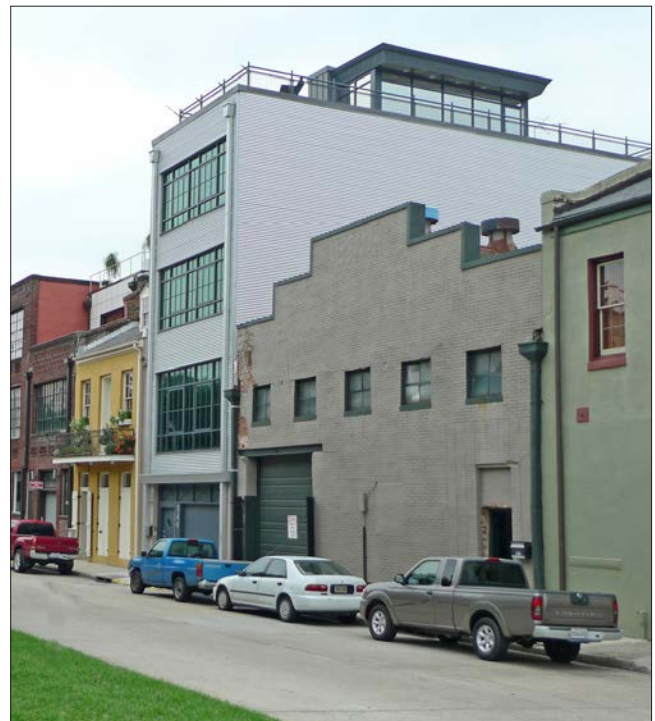
Corrugated metal, often used for garage doors in the Warehouse District, was used for the wall material at this new building.
