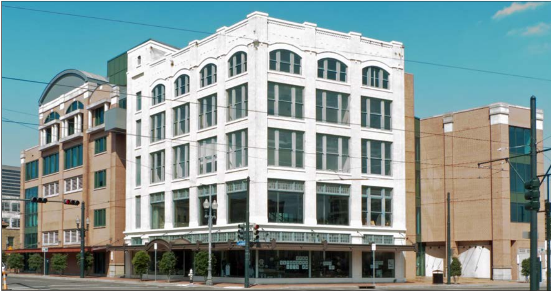
The additions to this corner building allowed the historic building to remain and be adapted for a new use.
