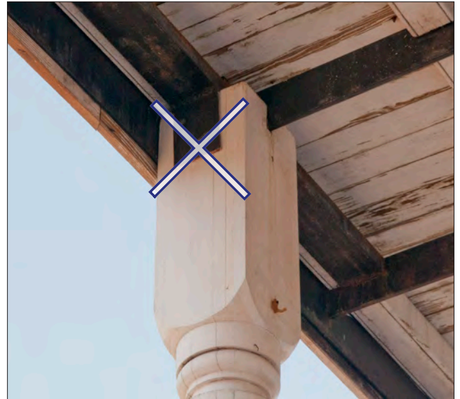
A hurricane connector can be utilized at the attachment of posts to the structure of a gallery or a porch. They typically require longer fasteners, such as nails and screws, than traditional connectors. To minimize their visual appearance, the connector should be painted to match the color of the material to which it is attached and not in a contrasting color, as in this example.
