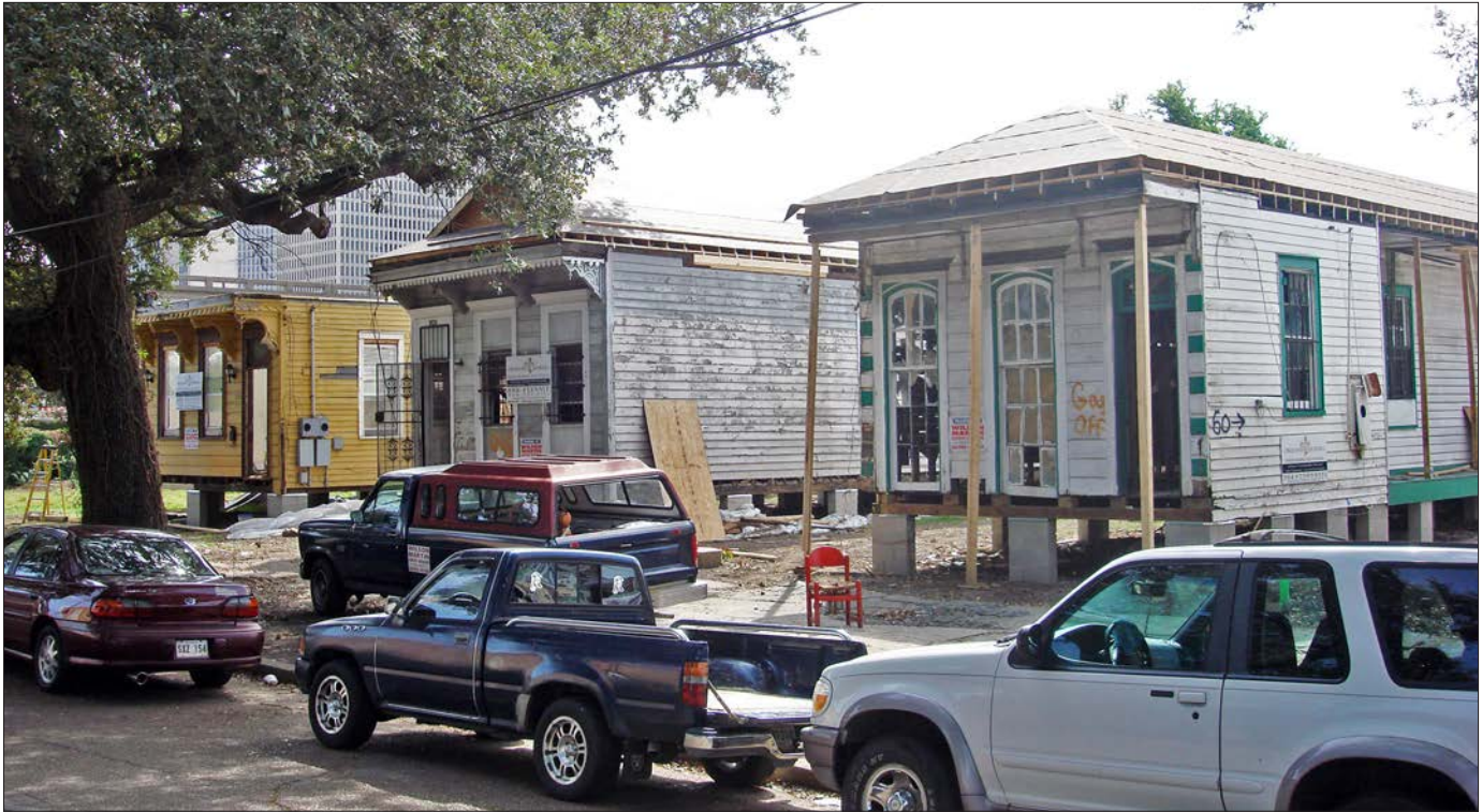
These Side Gallery Shotgun residences have been saved from demolition and moved to a new location. The entrance porches and roofs will be restored to prepare the homes for new families.
