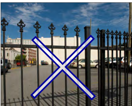
The fence around this parking lot has hollow metal pickets mounted to the outside face of the horizontal rails. Vertical pickets should be solid and pass through rails.
