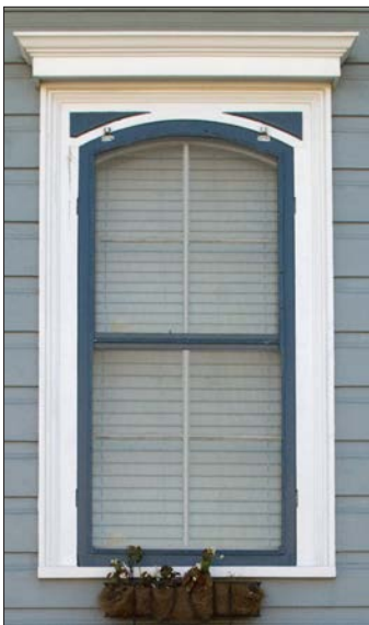
The arched wood screen fits the window opening.
