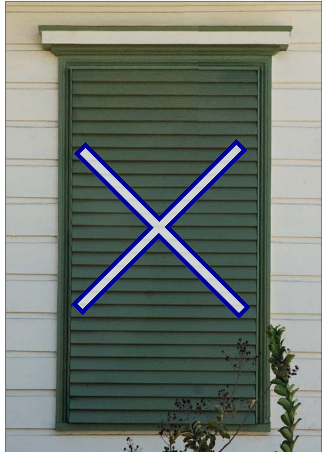
Hurricane shutters should not be permanently installed on windows. They should be stored and installed when needed for storms.
