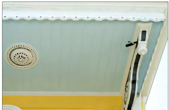
Security cameras, fans and lights should not obscure or be mounted to decorative elements such as brackets and soffits.
