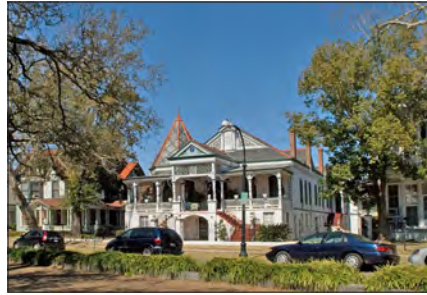
Esplanade Avenue is lined with trees and several grand homes
