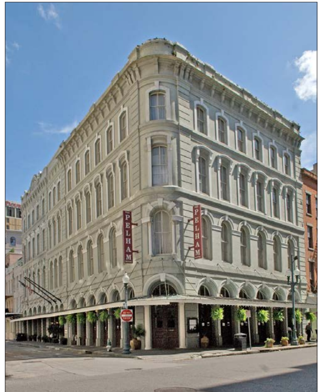
A flat or low-sloped roof is located behind the parapet and bracketed cornice.
