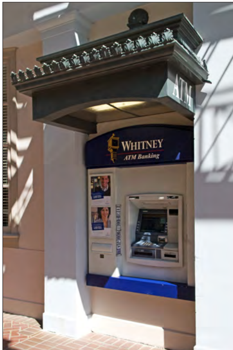
This ATM canopy was designed in a manner that complements the building's style and includes integrated down-lighting illuminating the immediate area.
