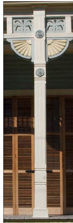
Chamfered Post with Brackets
