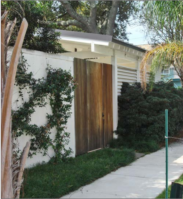
New secondary buildings should be complementary to existing historic buildings and the streetscape. This carport has a louvered side wall and roof structure with exposed rafter tails that resemble a neighborhood building.
