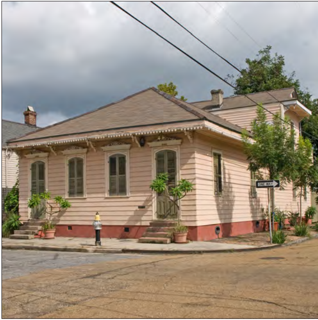
This Camelback Shotgun double has a deeply overhanging hipped roof over the main block and a side gable rear second story addition.
