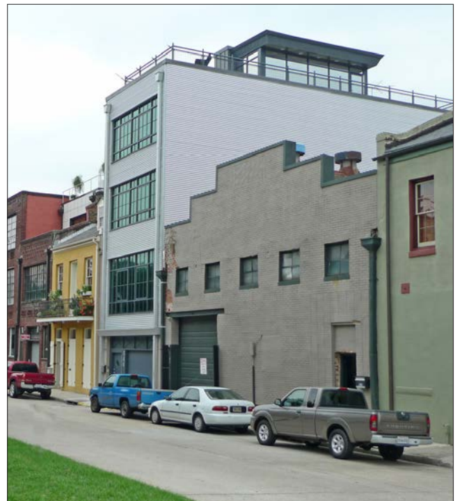
Corrugated metal, often used for garage doors in the Warehouse District, was used for the wall material at this new building.
