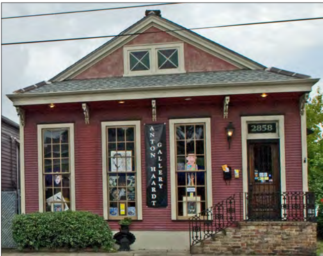
This former residence has been converted into a retail store.
