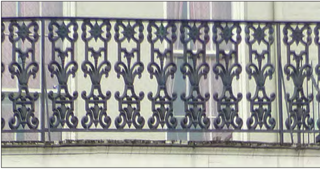
Cast iron decorative railings typically include a repetitive pattern of detailed components.
