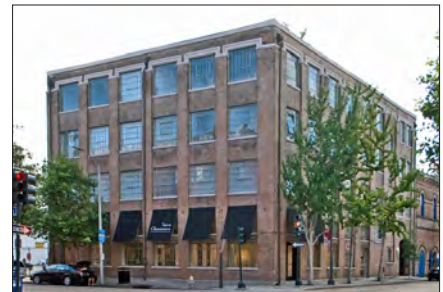
20th century buildings tend to be on larger sites and be more monumental in scale and design
