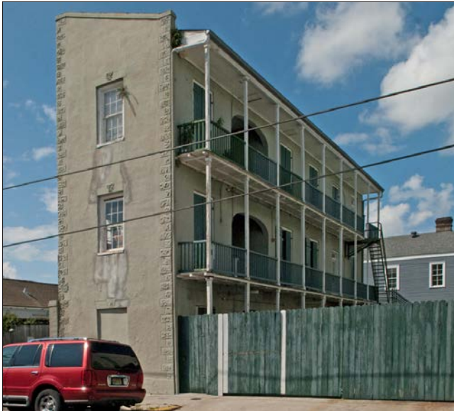
Secondary buildings can contribute to the streetscape.
