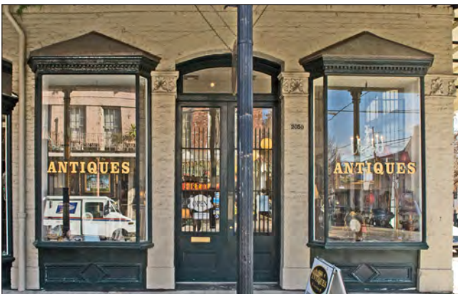
Vitrine windows flank the central entrance at this storefront.
