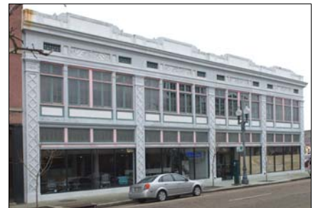
710 Baronne Street incorporates large storefront display windows
