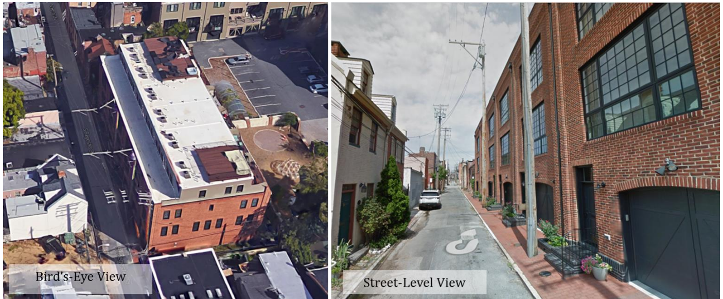
Figure 49. South Register Street between Aliceanna and Lancaster Streets.
