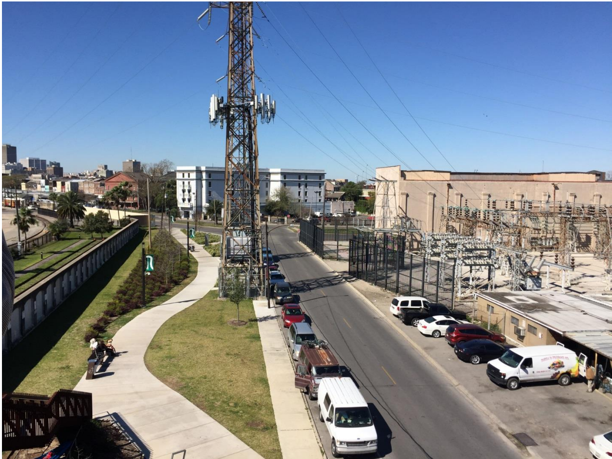
Figure 24 View from the Marigny entrance to Crescent Park towards Hotel de la Monnaie in the Marigny Triangle, which is five stories and approximately 55-60 feet in height.
