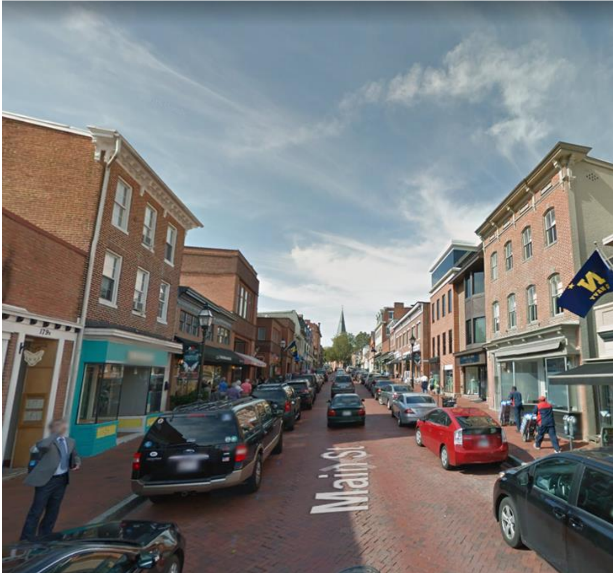
Figure 42. Views of Main Street within the Historic Annapolis Downtown Area. Height limits set at 45 feet on the left side of the street and 38 feet on the right.
