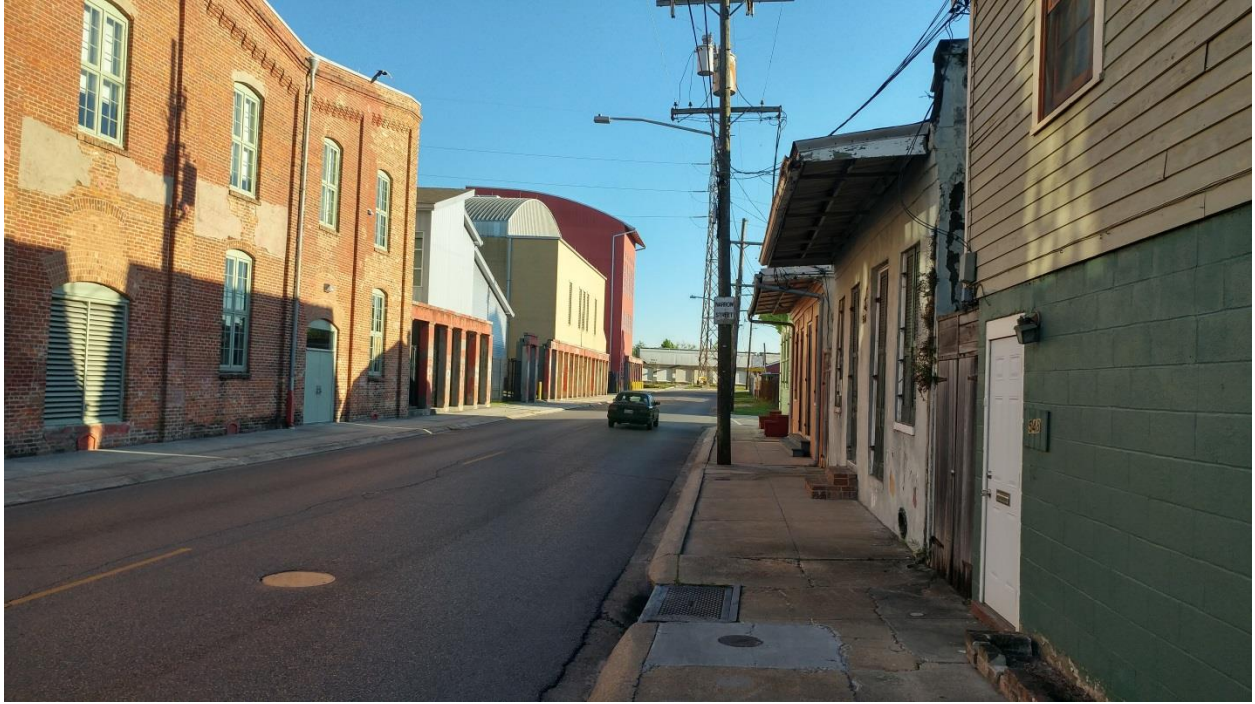
Figure 22 NOCCA buildings as seen from St. Ferdinand Street - 75 ft. portion of the building at the rear by the floodwall.
