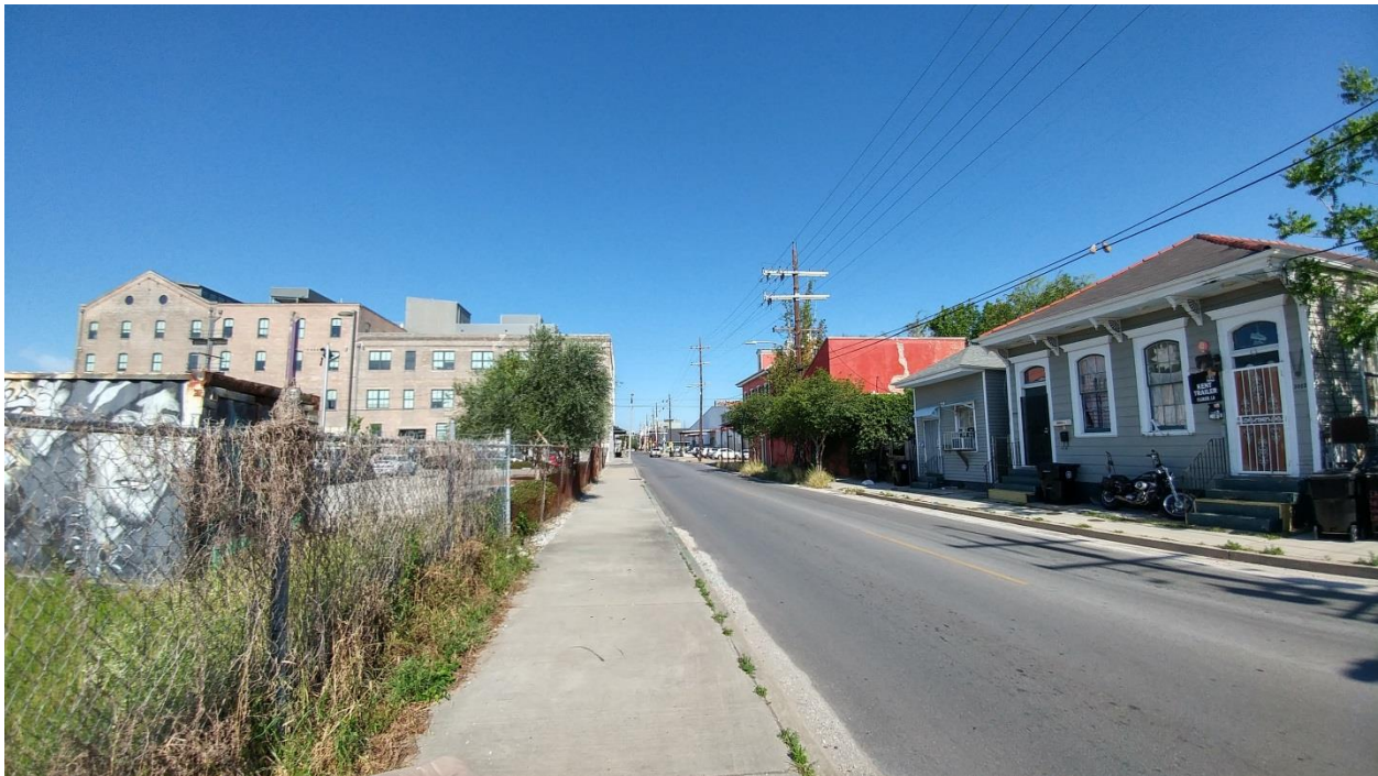
Figure 20 Chartres Street view with the Rice Mill and shotgun houses across the street one-half block away from each other. The Rice Mill's 75 ft. portion is at the left side of picture by the floodwall.
