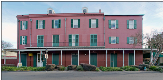
The use of brick and a simple, corbeled cornice is appropriate for this 1975 reconstruction of a French Market building.
