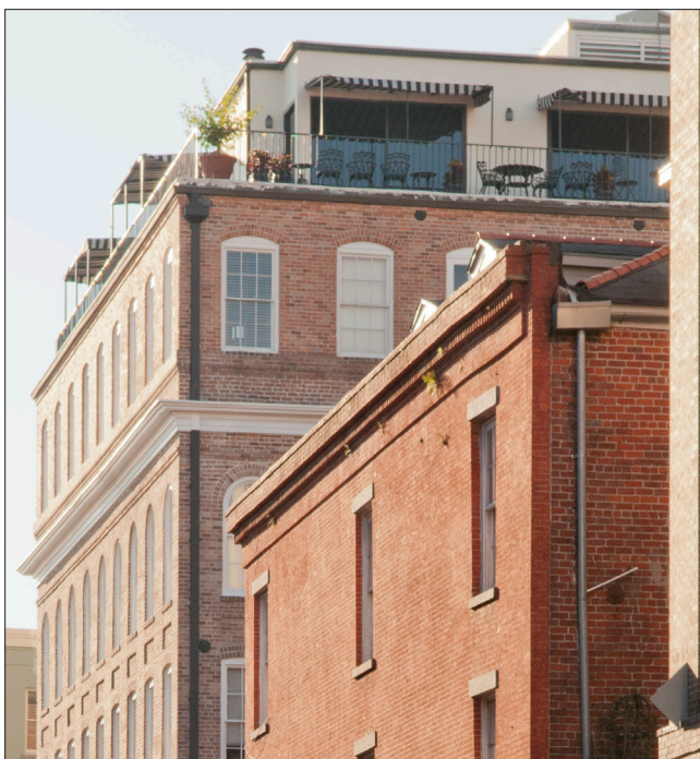
This rooftop addition is set back from the building corner on both sides and has a flat roof without permanent projecting overhangs. The metal railing is nominally visible to pedestrians.
