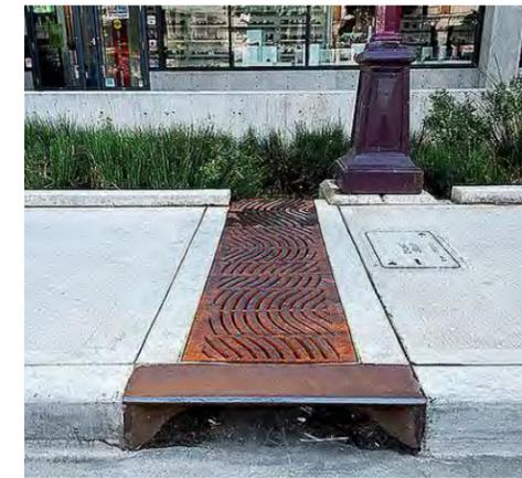
Grate connecting to street bioretention cells
